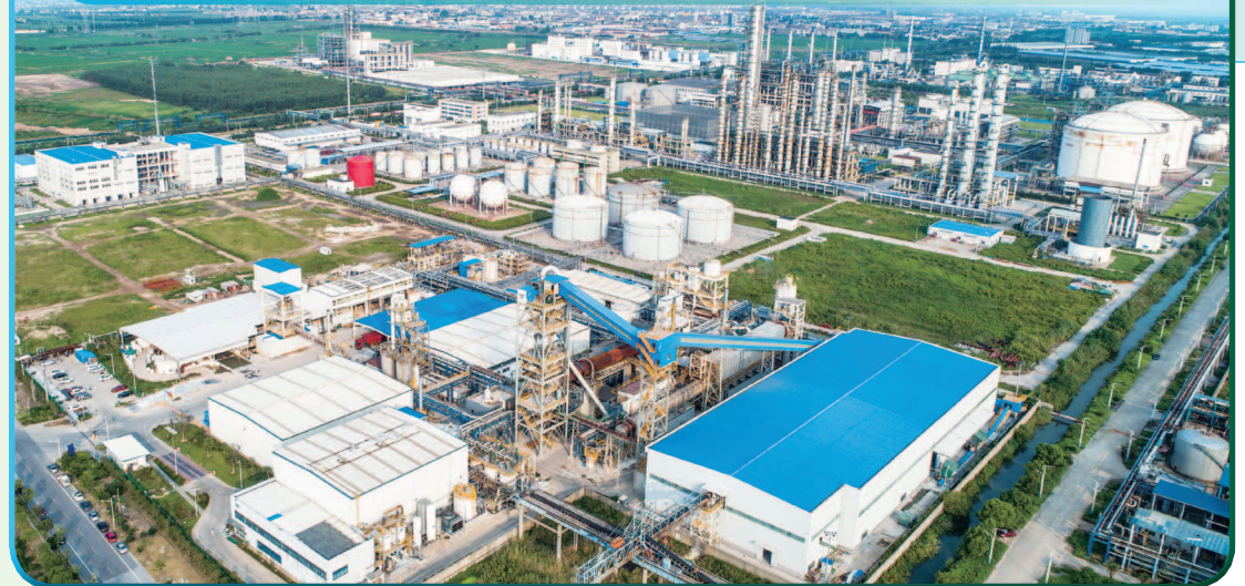
The Group supplies natural gas to this lithium battery material production company in Zhangjiagang, Jiangsu Province, for high-temperature roasting, evaporation, drying and other production processes.
