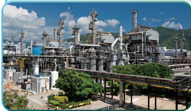
The gas production plant at Tai Po INNOPARK was commissioned in 1986.
